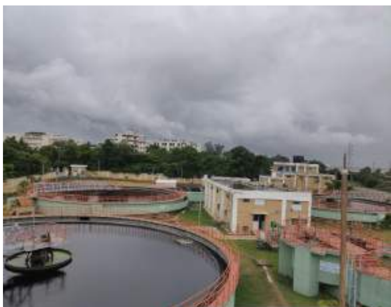
36 MLD STP at CDA-Bidanasi area of Cuttack
