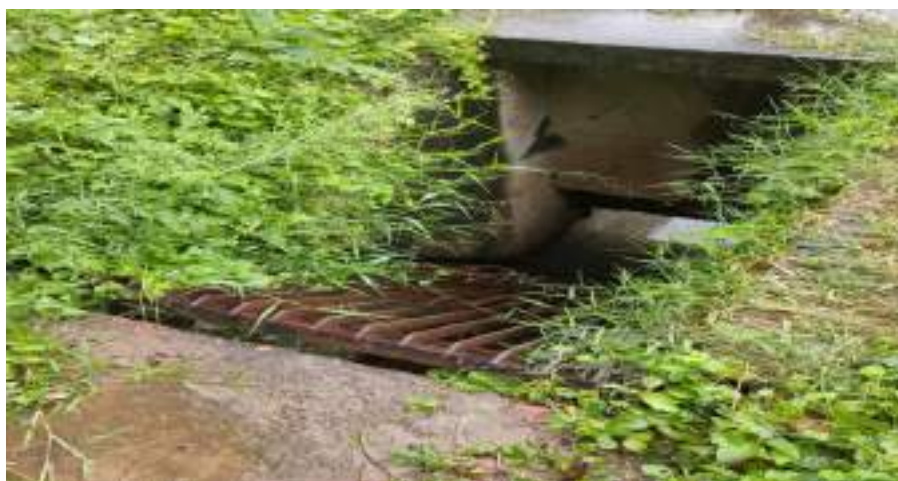
33 MLD STP at Mattagajpur Cuttack
