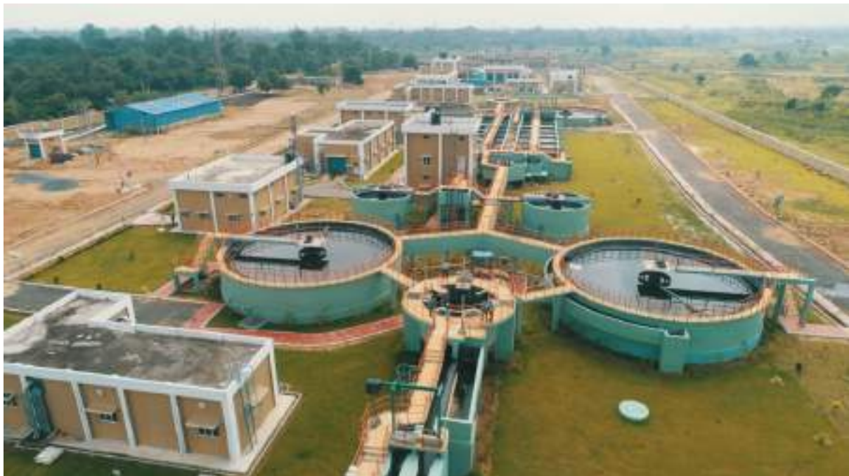
16 MLD STP at Mattagajpur Cuttack
